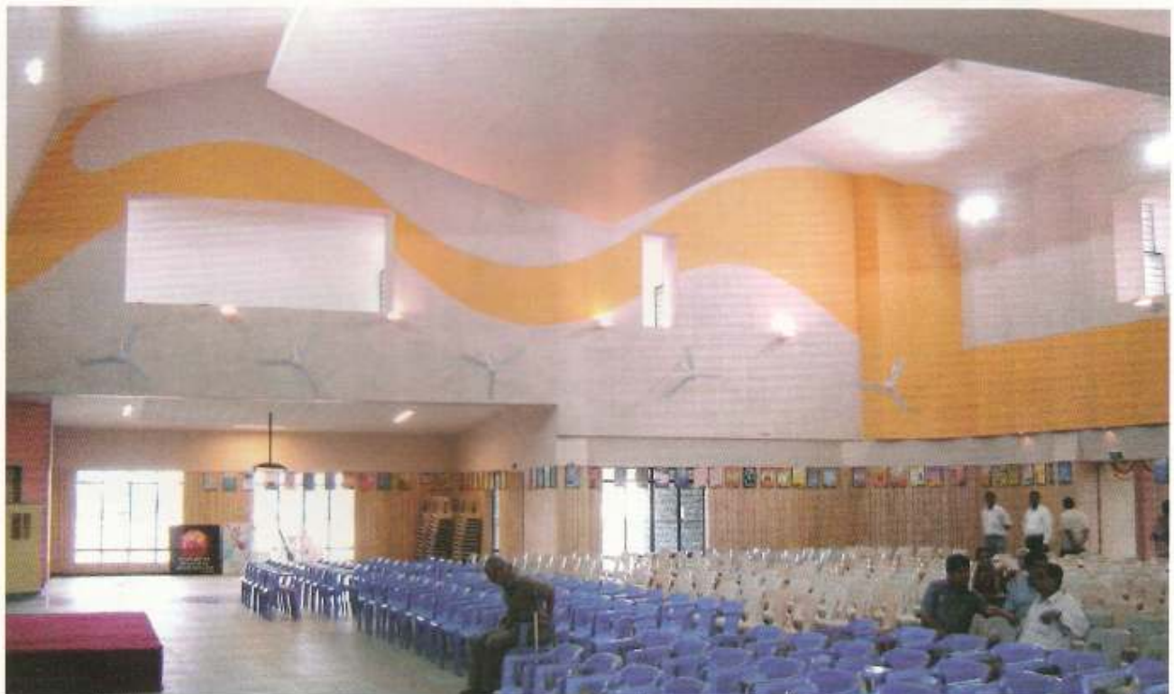
The auditorium in the school: Observe the roof pattern- an experiment in acoustics
